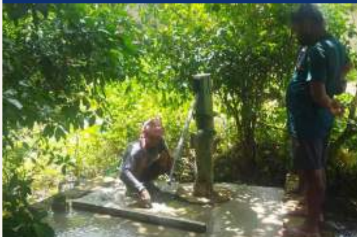
Renovation of Tube Wells
